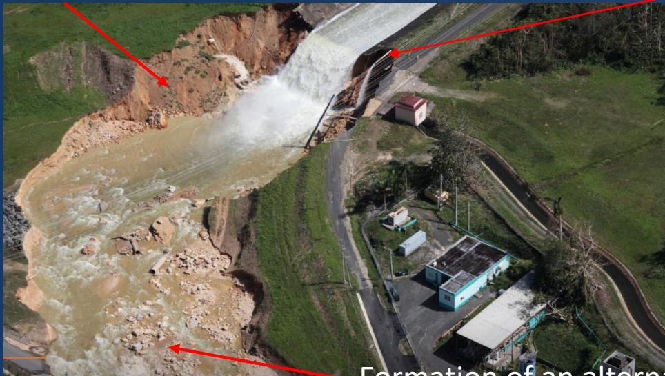
Formation of an alternative path for the water,, close to the dam
